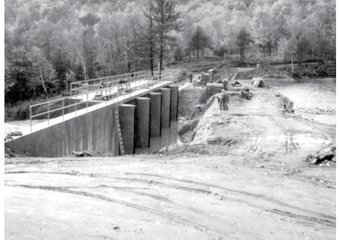
Dam being built in November 1966.
