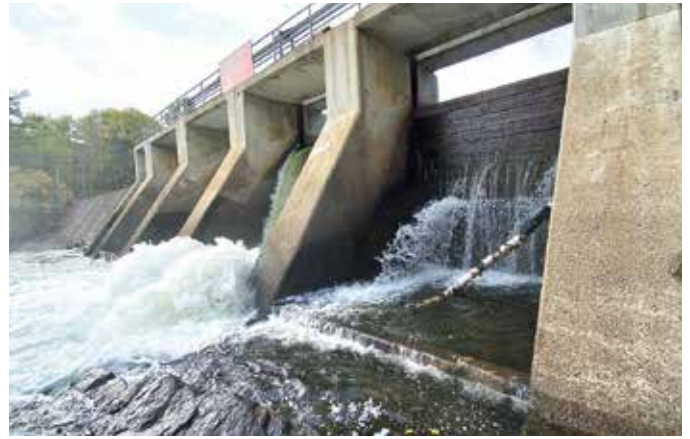
Side view of the sluices. Photo by MNRF
